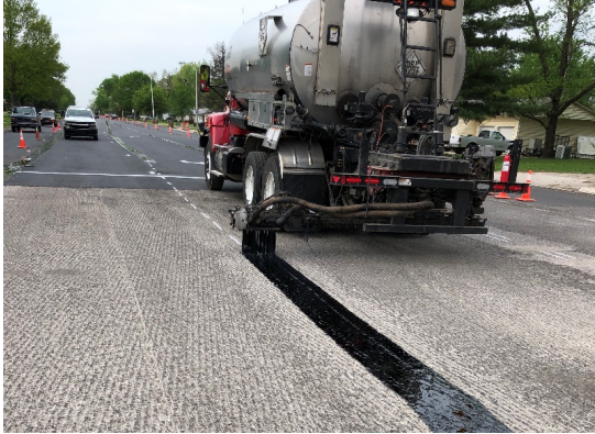
1 2 3 Figure 3 Heated pressure distributor and LJS spray bar 4
